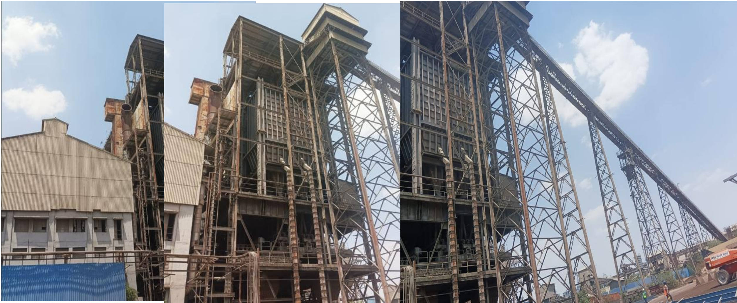
Thermal Power Plant (TPP-1) All mix material -MS, Rubber, SS, cables-all type, GI, Aluminum etc.)
