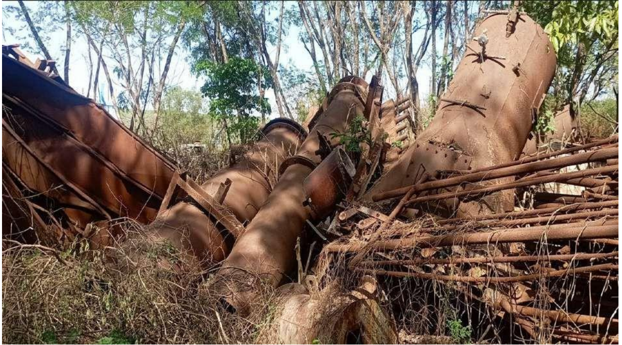
ESP scrap-MS structure
