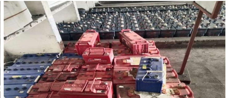
12. SCRAP HAZARDOUS - BATTERIES
