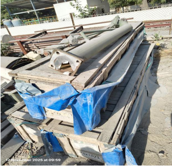
LOT 3 SCRAP POWER TRANSFORMER PART 2 CONSERVATOR
